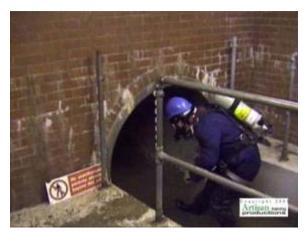
Combustible gases or vapors can accumulate within a confined space when there is inadequate ventilation. Gases that are heavier than air will accumulate in the lower levels of a confined space. Therefore, it is especially important that atmospheric tests be conducted near the bottom of all confined spaces.
