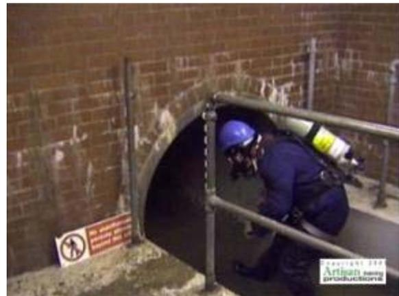
Combustible gases or vapors can accumulate within a confined space when there is inadequate ventilation. Gases that are heavier than air will accumulate in the lower levels of a confined space. Therefore, it is especially important that atmospheric tests be conducted near the bottom of all confined spaces.
